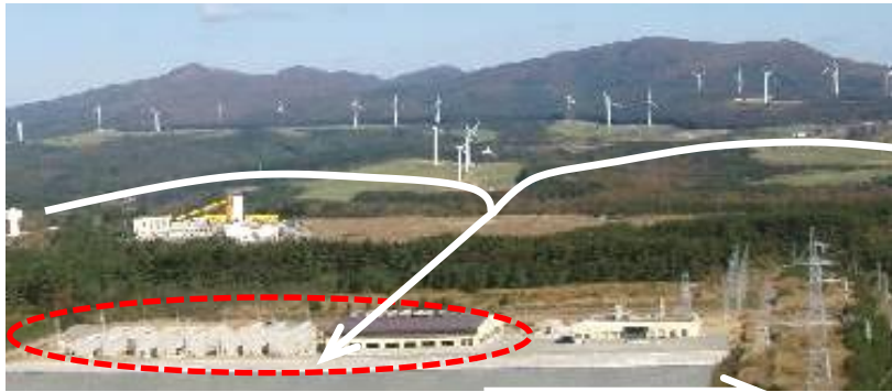
Battery Station (e.g. NAS Battery, 56MW/370MWh)
