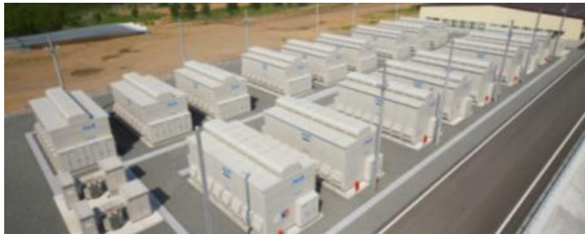
Battery Station (e.g. NAS Battery, 56MW/370MWh)
